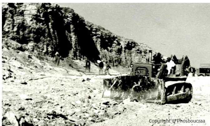
Fig 3.1: This image, from the Phosboucraa company page, shows some of the 1970s work at the mines. Source: OCP Online Company Archives.
